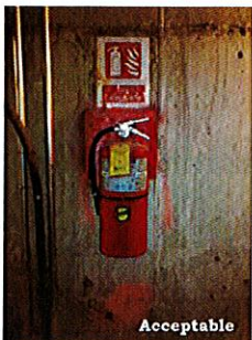
Fire extinguisher in a construction site.
